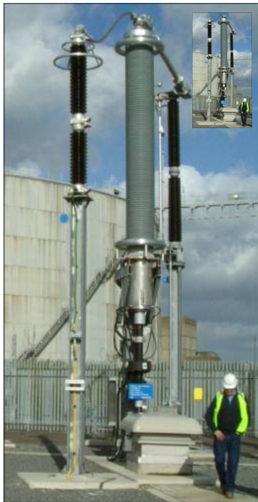
Figure 3 400kV Cable Outdoor Sealing End (ODSE) Termination
