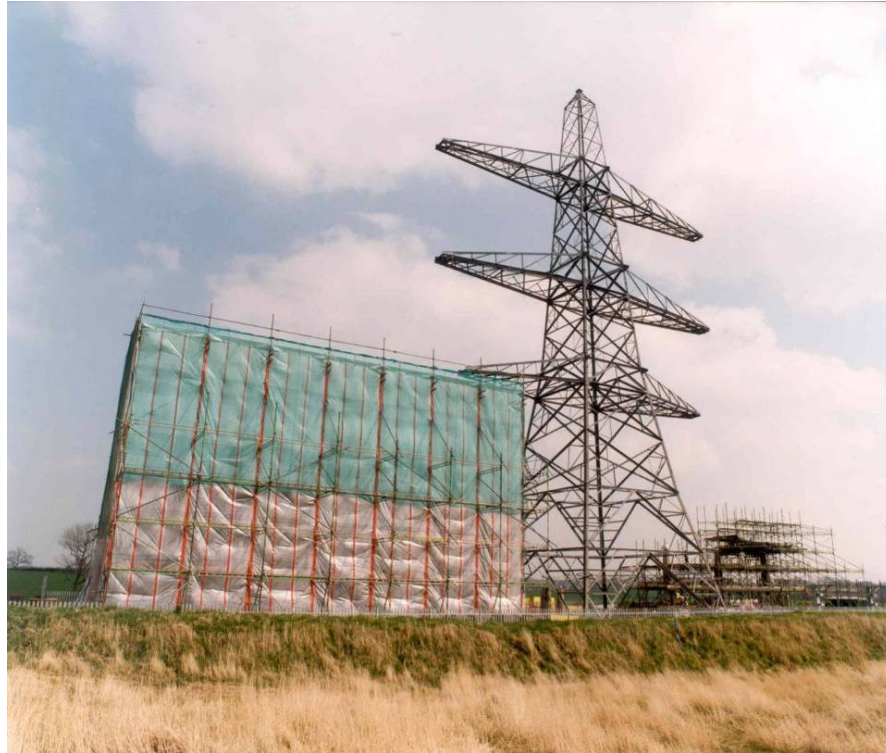
Figure 12 Weatherproof Sheeted Enclosure for Cable Termination Assembly
